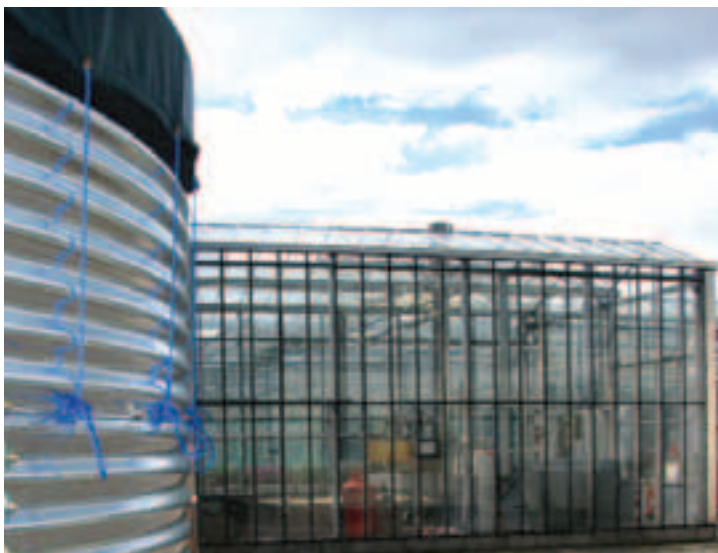
Fig. 7 Rain water harvesting installation at HDC, Greenmount Campus
