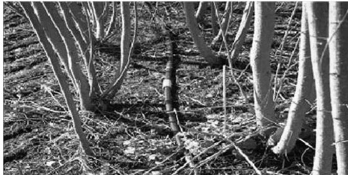
Perforated pipe for biofiltration of liquid effluent waste
